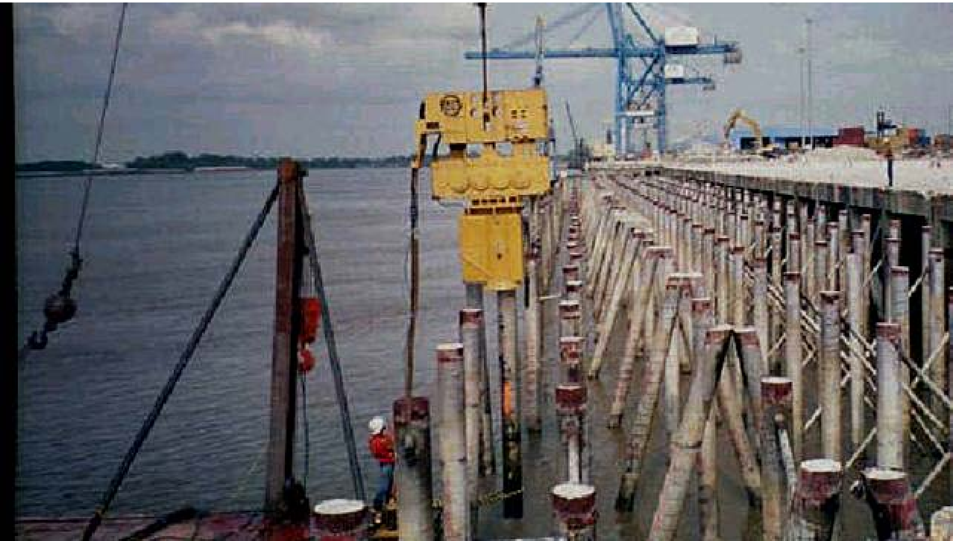
Example: Pulling Pile Piles
